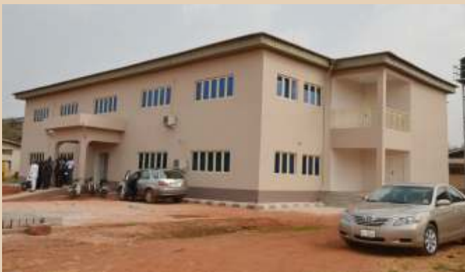
The NLNG-built and equipped research laboratory at University of Nigeria, Nsukka
